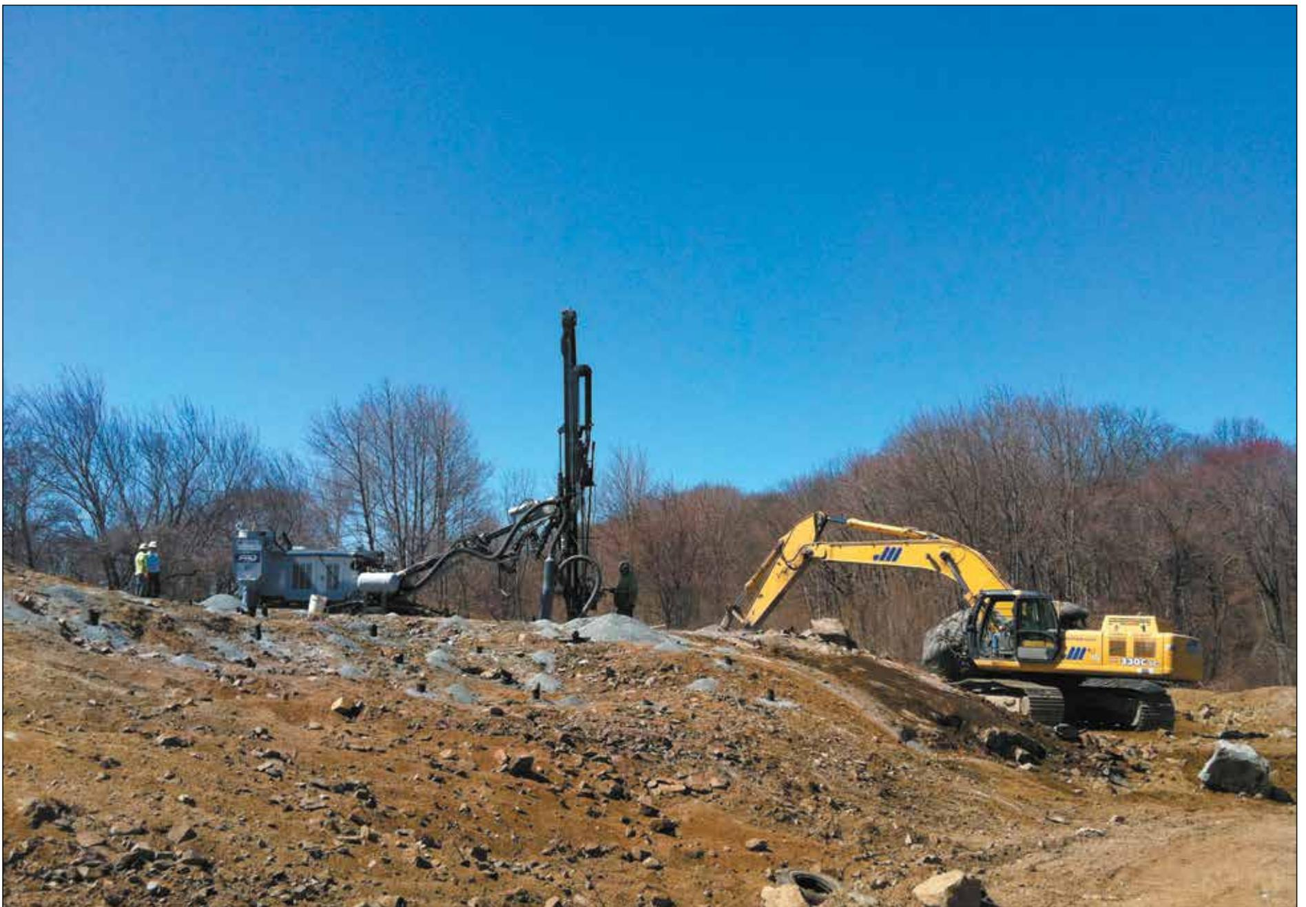
Overburden is removed by a Cat excavator as Furukawa HCR900 Track Drill bores holes for explosives.
