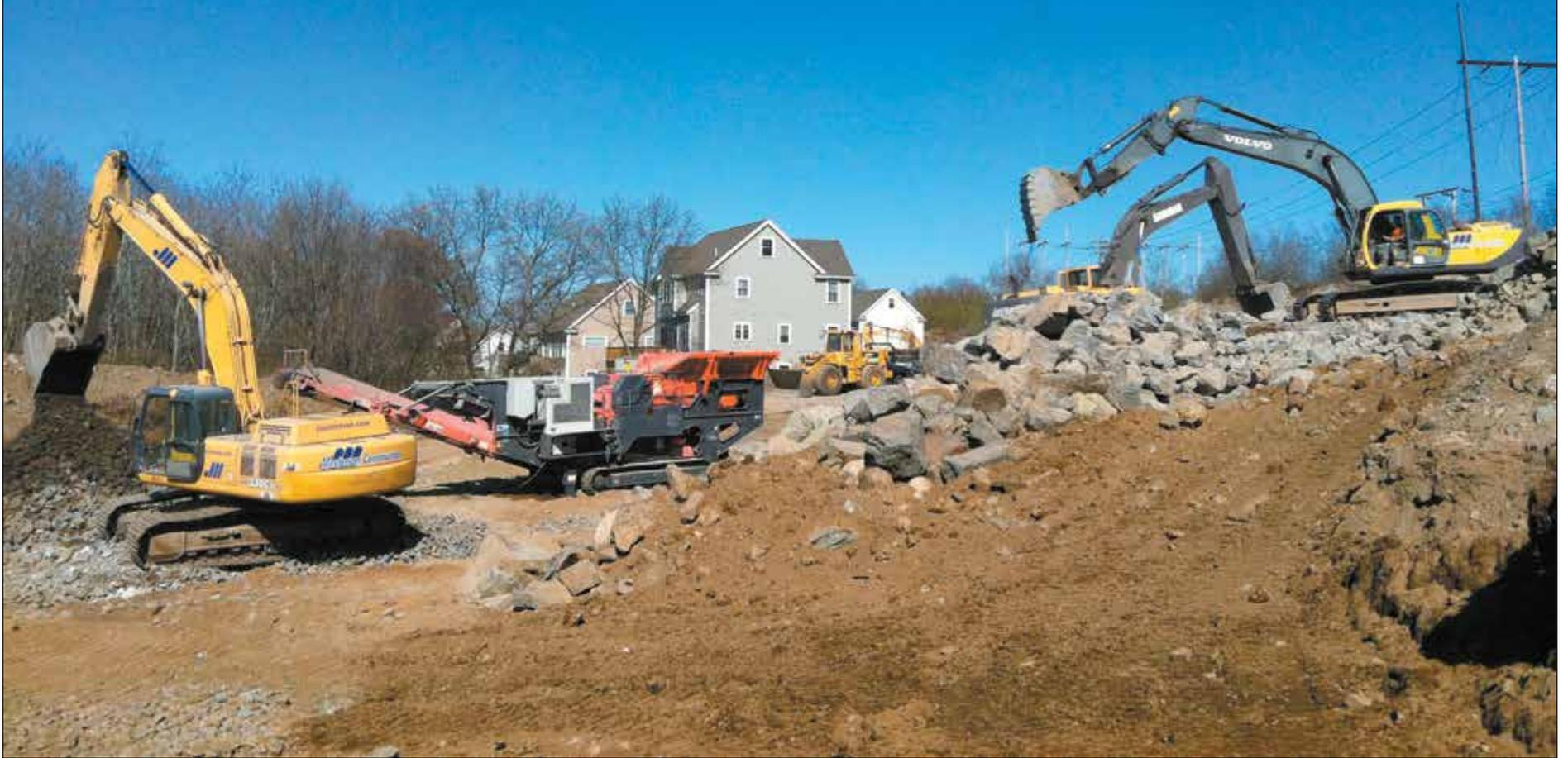
Working to clear blasted rock, from left to right, are: a CAT 330C Excavator, a Sandvik QJ341 Crusher, Akerman and Volvo excavators.
