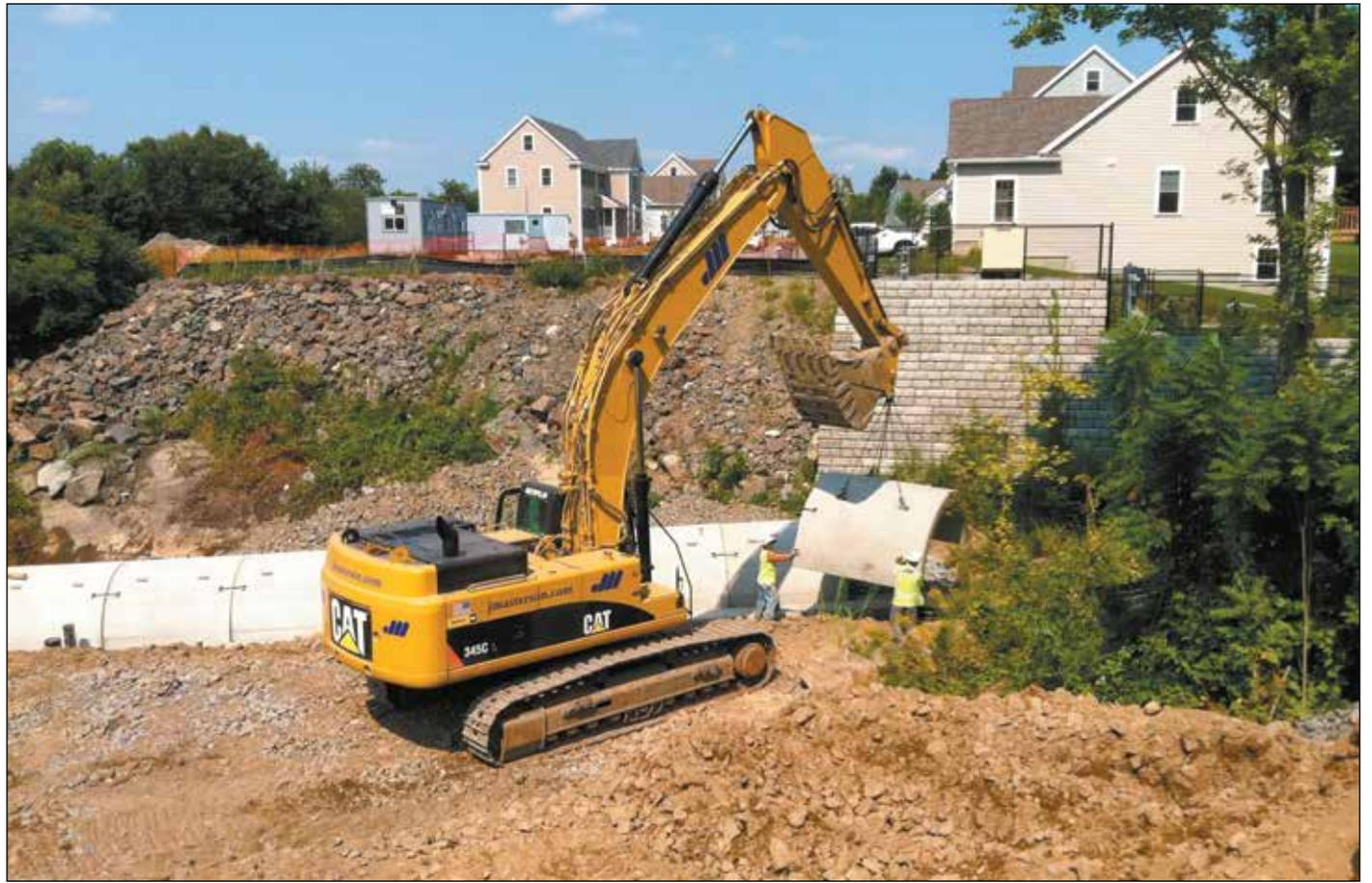
*A Cat 345C Excavator places Michie arch culvert section.*
